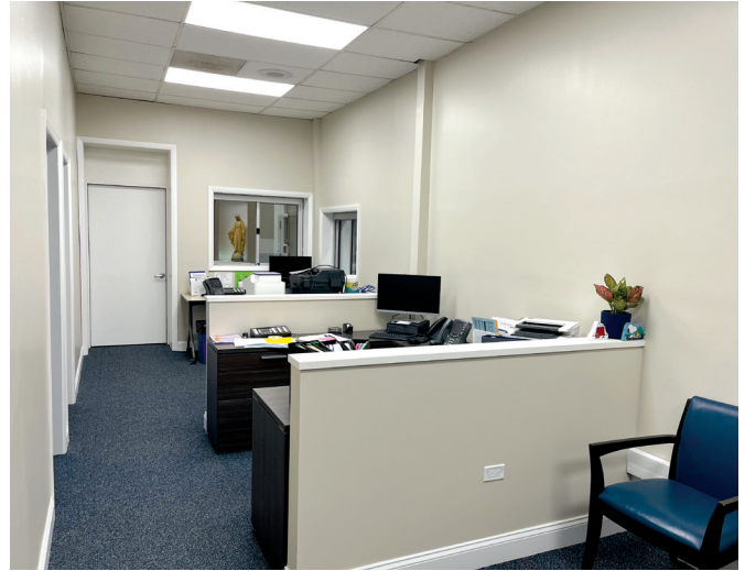
As of today, security door and security window are finished!
