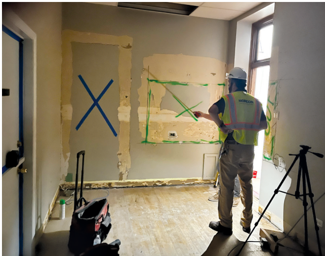
New security door and security window in the principal's office
