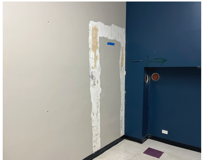
New office door being installed
