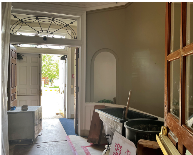
New security entrance in process as of Aug. 2.
