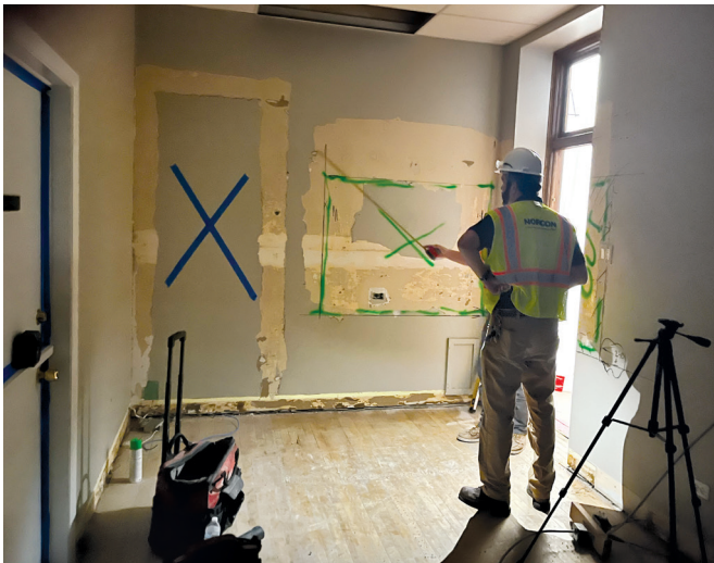
New door and window in the principal's office in process as of Aug. 2.
