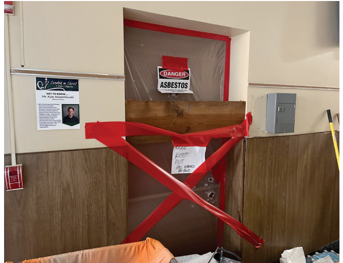
New elevator entrance
