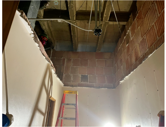
New elevator shaft being formed
