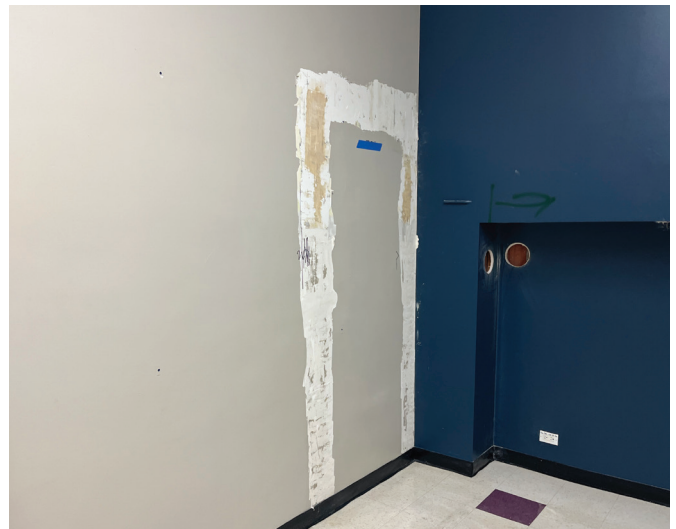
New office door being installed
