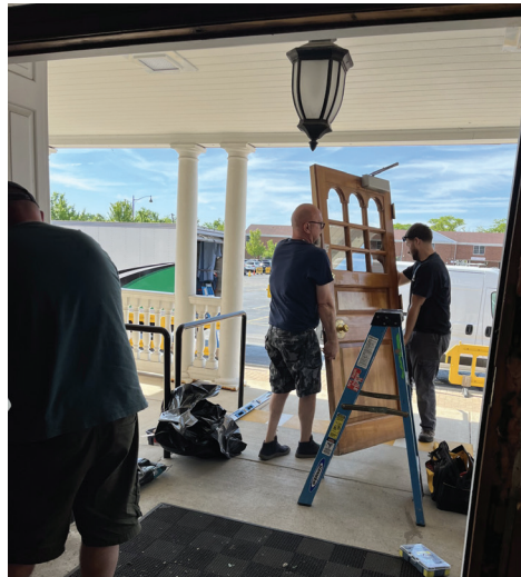
Old doors removed...
