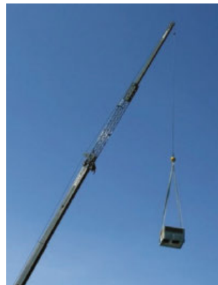
Air Conditioning components being maneuvered into place.
